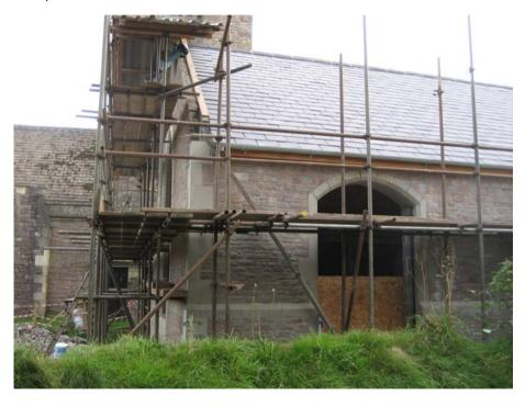
Mr Saysell has been working with the joiners who have measured the window apertures to enable the frames to be manufactured to fit stone clad apertures. Again this joinery work will be in keeping with the rest of the structure. All of this work is being carried out by craftsmen from the surrounding area.
